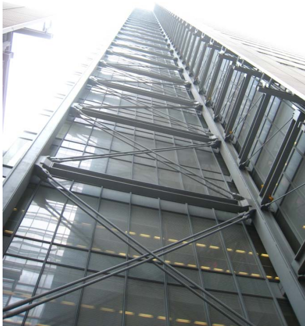
Figure 9: Exposed X-braced rods
