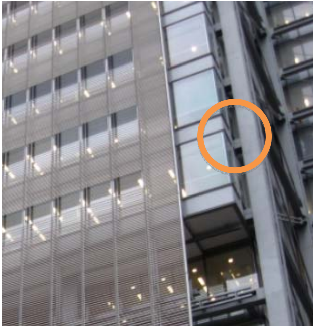
Figure 5: 'Dog-leg' beam connection
