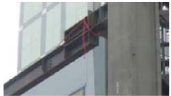
Figure 3: 'Dog-leg' beam connection
